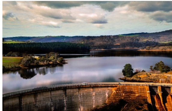
Myponga Dam (Australia)
